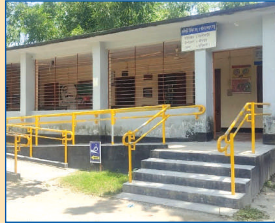
Ramp with handrails and even staircases implemented in a health centre of Sitakund Upazila accessible © HI
