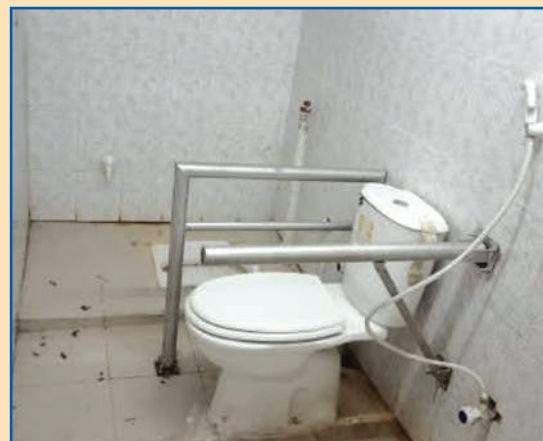
Door could open from inside, electric switch board placement was changed and high commode with handrail installed making a health centre toilet of Sitakund Upazila accessible for person with disabilities © HI
