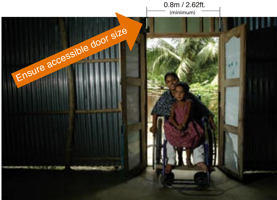
Accessible house with proper door size
