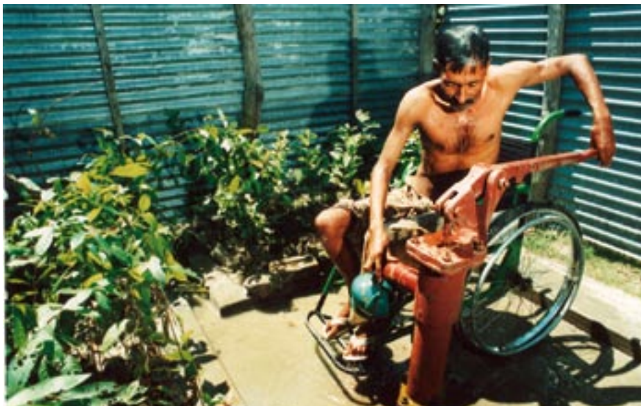
Accessible Tubewell with small steps and slope to platform
